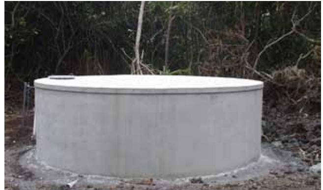
Ferrocement tanks, also known as ferrocement tanks, are new to the local market and growing in popularity. Like solid concrete tanks, they can be designed into a home's structure.
