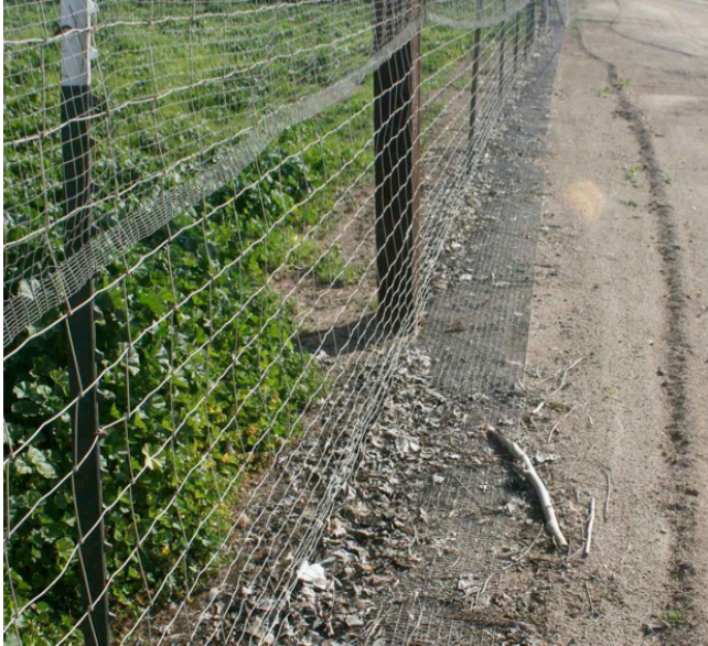
Figure 8. Example of woven “hog wire” exterior fence with a cage wire skirt to prevent digging under. Others will use barbed and/or electric wire along the bottom to prevent burrowing.
