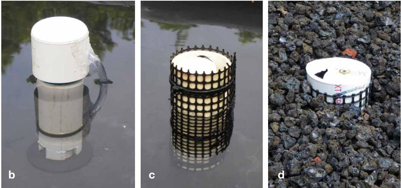
**3b-d.** The bottom of the bell cap is even with the height of the standpipe, and thus with the desired water level. This level should be predetermined so that when the gravel guard is installed (center) and the medium is added (right), the water level is 1–2 inches below the surface of the medium.
