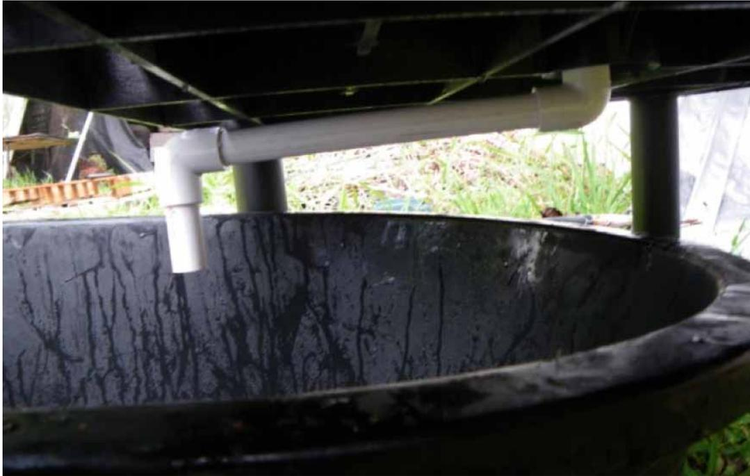
**16.** The drain assembly on the underside of the grow-bed. Note the two sequential 90° elbow fittings, which help start and stop the siphon and direct the flow of water back to the rearing tank beneath the grow-bed.
