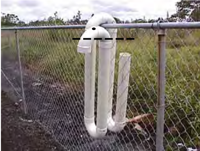
An overflow device to keep the water level as indicated by the dashed line. Pipe on the near side of the fence hangs outside the tank. A hole atop the elbow in the foreground is needed for proper function, but if a T-joint is used, the hole is not needed.
