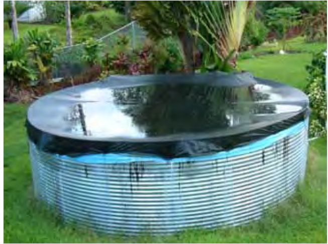
Mesh covers often sag into the water when the tank is full or the mesh stretches in the sun. The resulting puddle attracts birds, insects, and debris, which contaminate the water.
