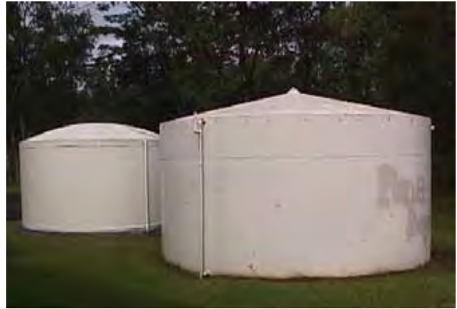
These enclosed metal tanks are well maintained on the outside, but problems may arise if there is deterioration on the inside.
