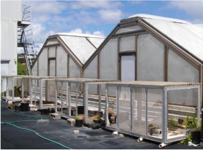
The greenhouses on the top of Gilmore Hall are to receive air conditioning once a new power line is in place.
