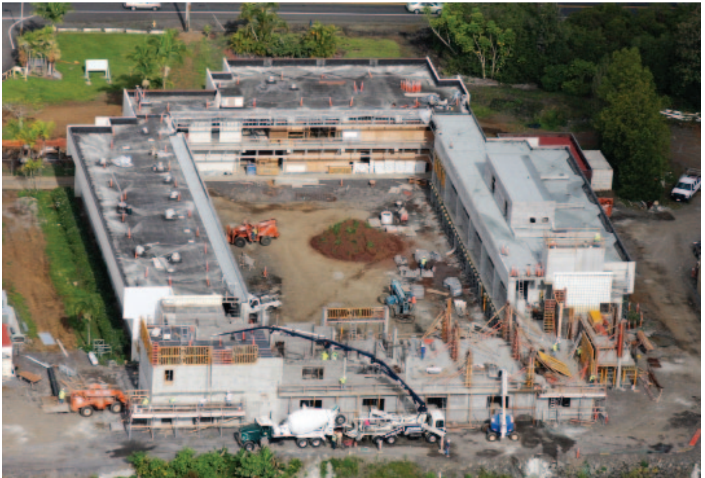
What Komohana looked like when work was in progress.
