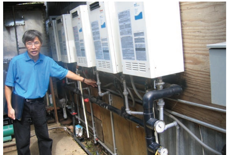
Dr. Marcel Tsang inspecting tankless water heaters installed to provide hot water to a freight container converted to a hot shower chamber at Leilani Nursery in Waimanalo, Hawaii to treat potted plants from the Big Island.
