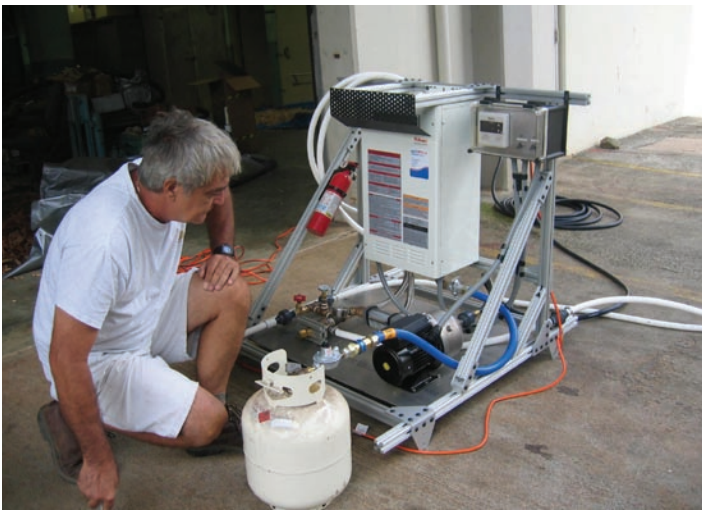
Charlie Nelson checking the instant water heater used as a source of hot water for the shower chamber.
