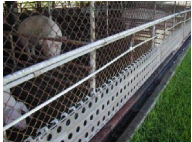
Concrete manure collection gutter outside pens
