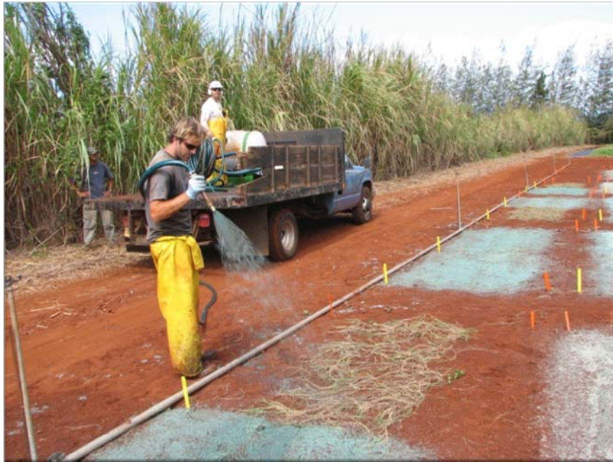
Figure 2.5. Application of hydromulch over cut stems of S. virginicus .
