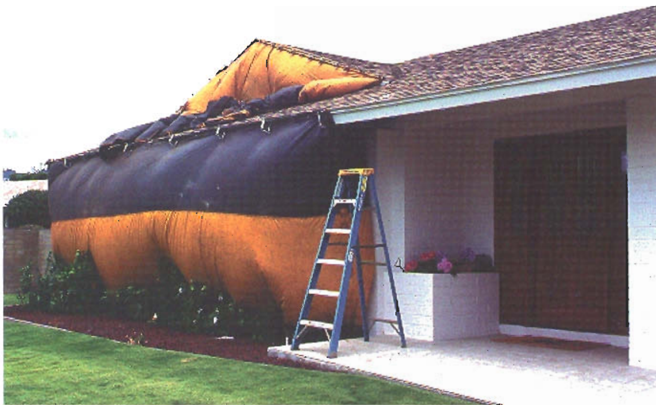
Unlike fumigation, TPE is typically done in a spot-treatment fashion and does not require that the whole structure be covered.
