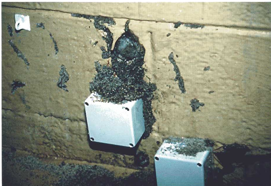
Fig. 4. Bait stations hot glued to elastomeric wall covering in a larval holding room.
