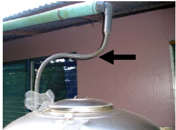
The arrow points to an area in the piping that allows water to stagnate, resulting in bacteria growth and poor water quality.
