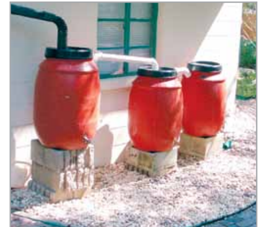
Multiple barrels provide for greater water storage.
