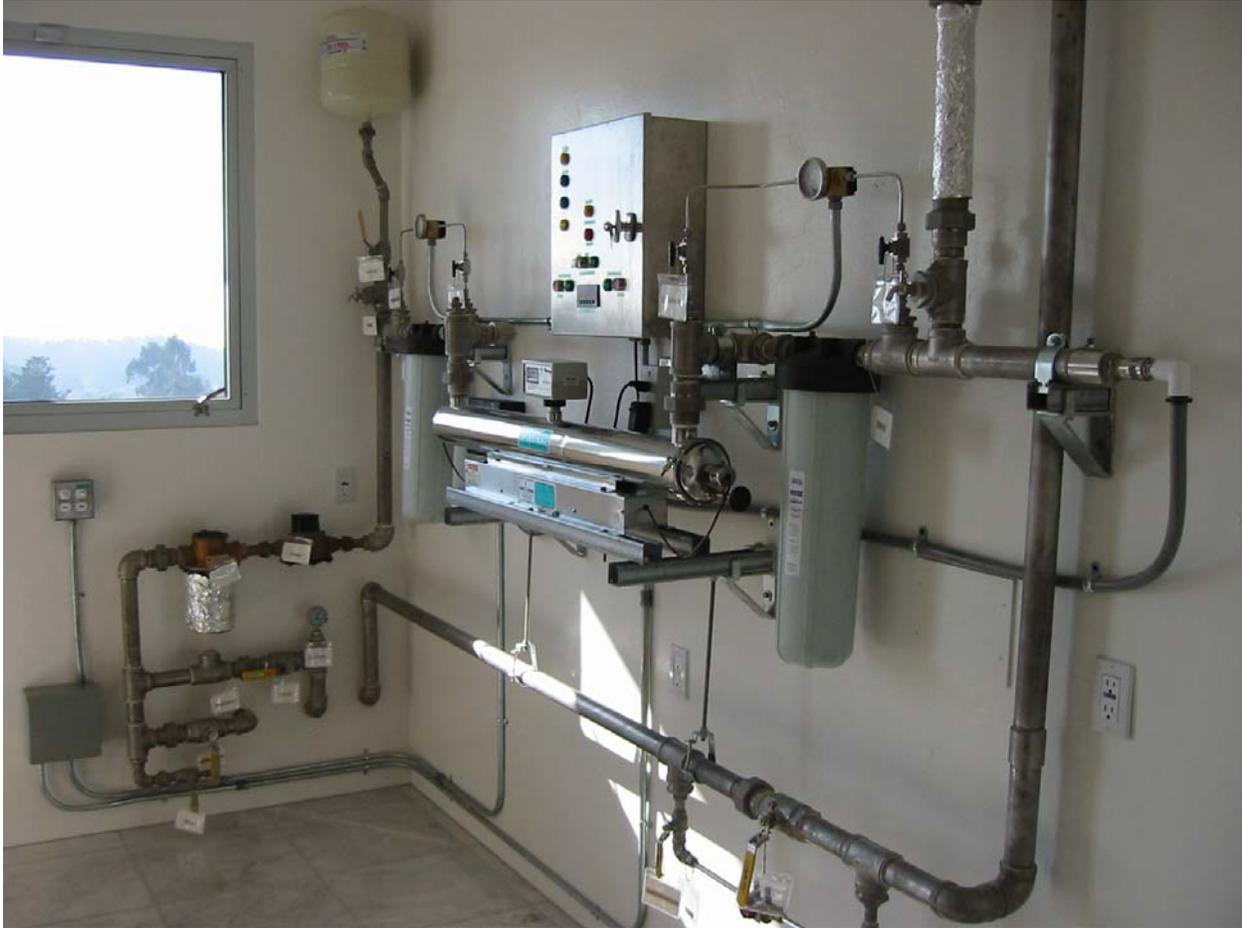
Filtration/pump control room. From left to right, inlet strainer and water flow meter, expansion tank (above), pressure transducer and pump control unit, cartridge filter, ultraviolet disinfection lamp with ultraviolet light monitor, 2<sup>nd</sup> cartridge filter, connection to domestic water distribution. Stainless steel square control box. Recirculation connection back to underground cistern.
