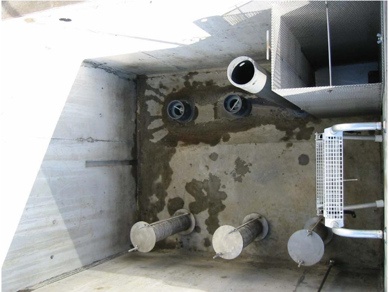
Roofwasher/filter vault. From top left to bottom right, flotruie rainwater diverter valves (2), overflow, leave basket, inlet filters (3), access ladder
