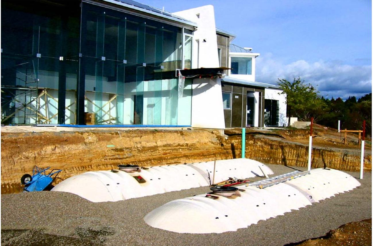
Rainwater Cistern (two 20,000 gallon cylindrical tanks) being backfilled with pea gravel to prevent empty tanks from floating during ground water saturation
