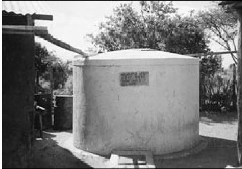
Figure 2: Ferro-cement storage tank (capacity 3200 liters).
