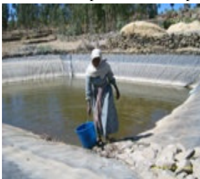
Figure 4: Trapezoidal pond blanketed with plastic sheet (Photo Ababi T.H, 2005)
