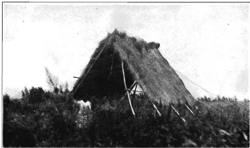
FIG. 2.—GRASS THATCHED SHED FOR CURING PIGEON PEA HAY. PROTECTS FROM RAIN BUT ADMITS FREE CIRCULATION OF AIR.
