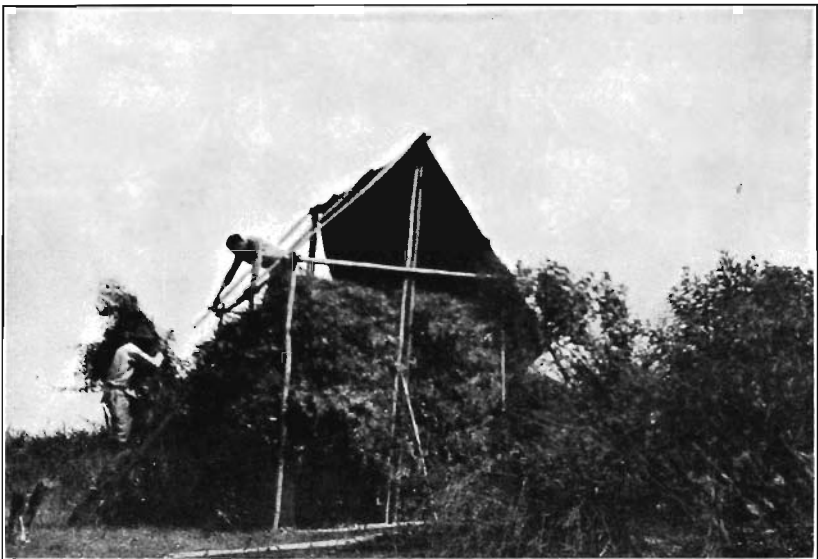
FIG. 2.—PERMANENT CURING SHED 8 BY 16 FEET. BUILT OF BAMBOO POLES WITH ELEVATED PLATFORM. CAPACITY ABOUT 2 TONS CURED PRODUCT. COST ABOUT $5.
