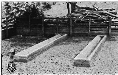
FIG. 14.—V-shaped concrete feeding troughs. Sanitary and durable.
