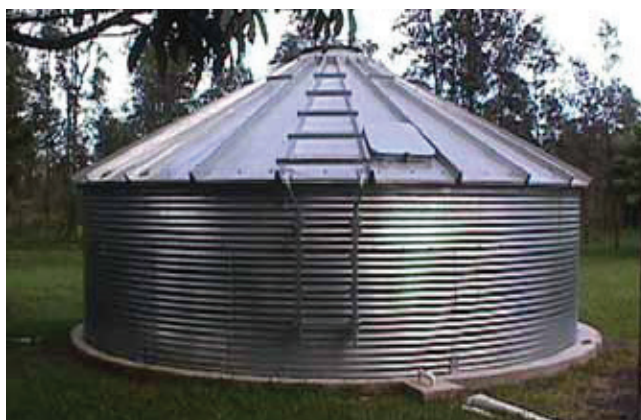
Some corrugated tanks have solid covers. This model has a top hatch for access and a liner secured to the sides with bolts.
