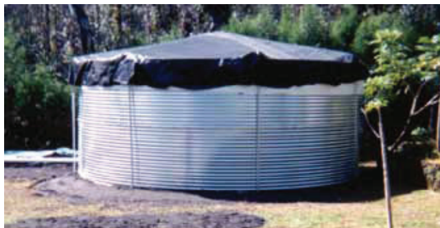
Pipe arches supporting a mesh cover keep it from sagging into the water.
