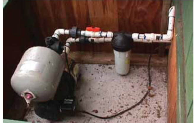
A small but typical electric pump. The pump sits below a pressure chamber. A coarse filter hanging from the inlet pipe filters the water before it enters the house.
