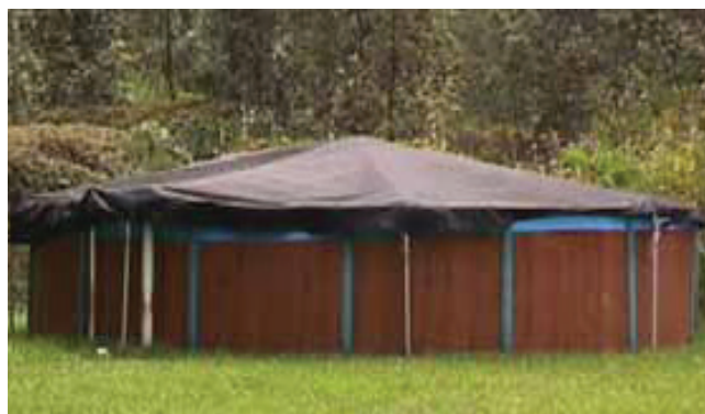
A large swimming pool tank with pipe arches holding up a mesh cover. These tanks are popular for their price and ease of assembly.
