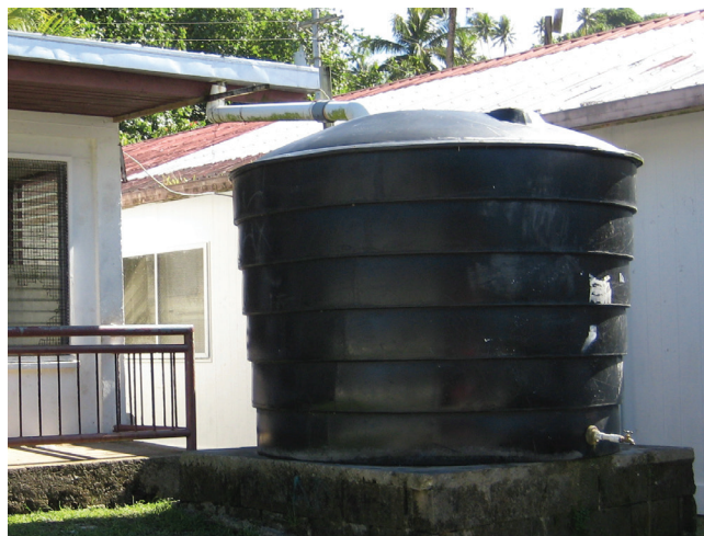
The U-shaped downspout-to-tank configuration at left is typical but undesirable. The pipe runs down from the roof, across the ground, then up and over the tank. Between rains, water is left standing in the pipe. In the system at right, the downspout is completely drained by gravity.
