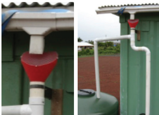
Homemade leaf screens and first-flush diverters can be made inexpensively, such as this one, which uses a large funnel and galvanized screen to keep leaves out and PVC pipe to divert the first flush of water.
