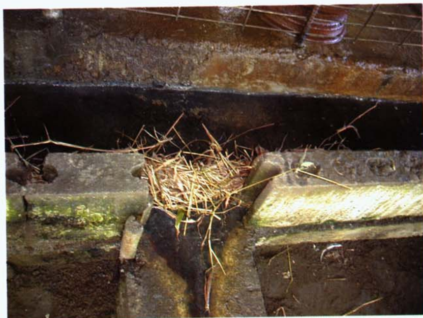
Grasses help filter out larger pieces of manure that would clog the holes in the rain gutters.
