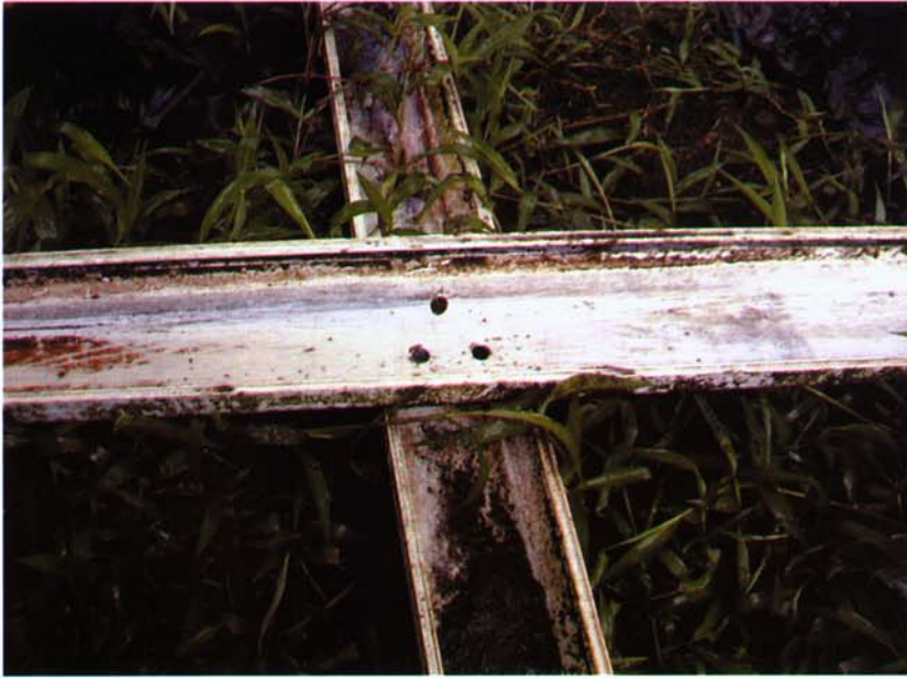
7. For crossover connections, drill several holes for the wastewater to flow through.
