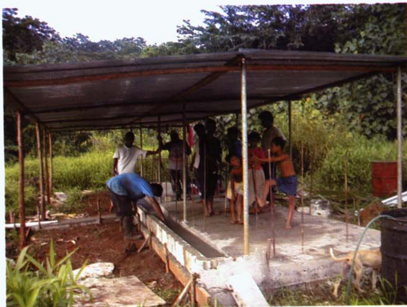
A concrete pig pen with a concrete gutter along its side. The wastewater flows into the gutter and from there to plastic rain gutters that fertilize the plants. Solids are filtered out (see below).
