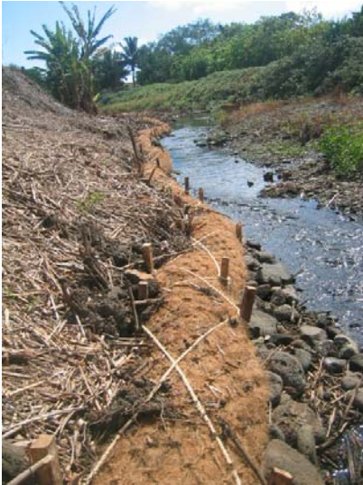
Coir rolls at Saddle City stream restoration site
