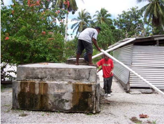
Fig: 6-Measuring the Height of Water.
