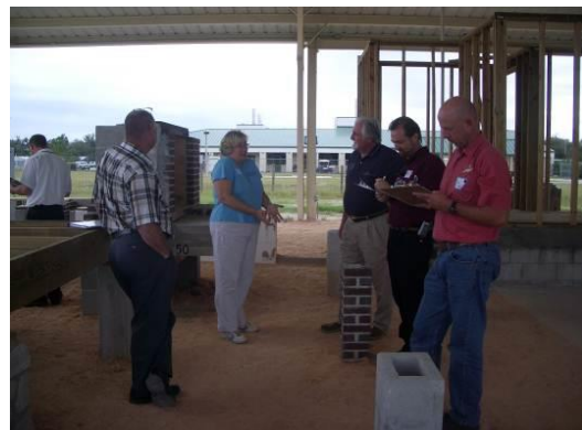
Fig. 4. County faculty Pam Mattis leading discussion on treating various piers
