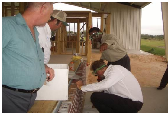
Fig. 3. Exercise to teach concrete patching after drilling for liquid termiticide application
