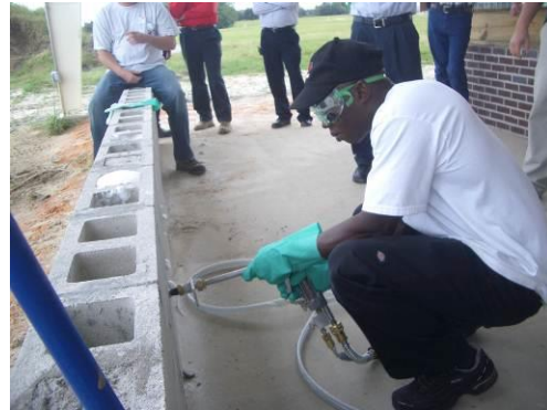
Fig. 2. Practice foaming wall voids according to pesticide label directions
